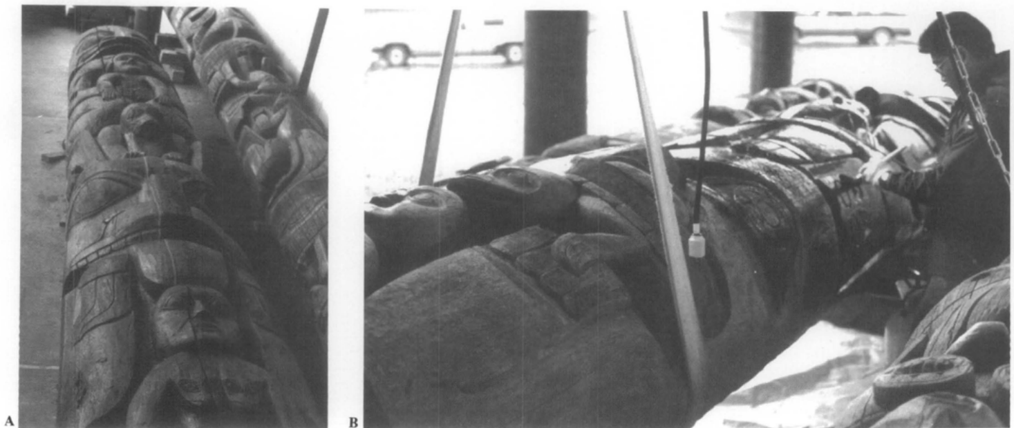
Figure 7. Borates were applied to the totem using a garden sprayer and brushes. This was followed by an application of a water repellent with mildewcide. Photo A is during application and photo B shows totems while drying.
